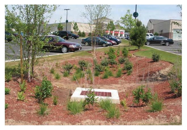
Figure 4.1. Bioretention in parking lot (photo credit: Center for Watershed Protection, Inc.).
