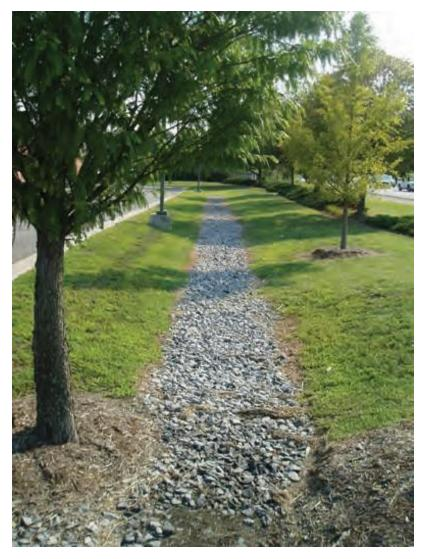
Figure 4.16. Infiltration practice in median strip.
