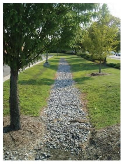
Figure 4.16. Infiltration practice in median strip.
