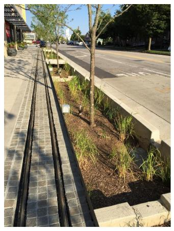
Figure 4.5. Example streetscape bioretention.
